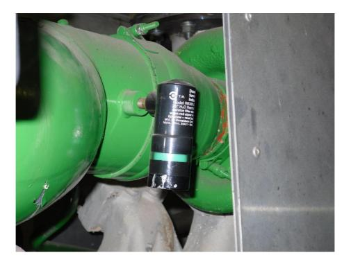
Above the batteries hidden slightly behind a metal plate is an air intake suction indicator. There is one on both sides of the generator to be checked. It can be seen in the picture the band inside the indicator should be *green* indicating the airflow into the generator is good, if this turns *red* then the air filters will need replacing by Dale Power.
