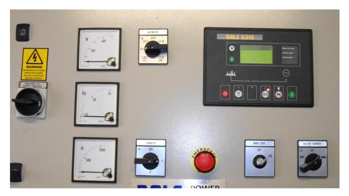
This is the main control panel mounted on the end of the generator. The display on the Dale 5310 should show 'Waiting in Auto'. If any errors are shown, the book on the controller is located on the bookshelf to the right of the shift leader's desk, or the support provider, Dale Power Solutions, should be informed. The Auxiliary AC supply switch on the left hand side of the panel should be ON, the Battery Charger switch on the Right hand side should be set to Normal, and Mode Lock should be ON.
