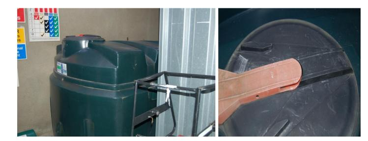
The 2000 Litre fuel tank is situated at ground level under the generating set. To check the fuel level, pull the lever and twist the top. There is no gauge for this tank so visual inspection of the fuel has to be carried out.
