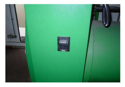
To the right of the control panel on the side is the main generator output switch; this should be in the up position as shown.
