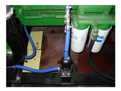
Next is the other water heating / pump device, check for leaks and the black handled valve above should ALWAYS be in the open position, there is also another black handled valve to the left of the pump just visible in the picture above. This is also a good advantage point to check under the generator for leaks on this side of the generator.
