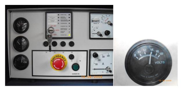
The control panel checks consist of making sure the green power on light is on, the key switch is in the AUTO position, and the battery Volts (lower left gauge) shows 13.8V as this shows a fully charged battery.
