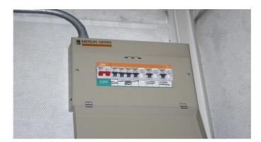
The location of the distribution board is in the corner of the generator cabin. All circuit breakers should be in the 'on' position.
