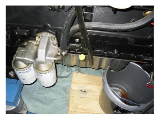
This is the other side of the generator. The yellow is the top of the dipstick. It can be seen in the middle of the picture above. This is just pulled out and the oil level should show, be on the upper notch of the dipstick. The bucket is to catch diesel fuel that seeps from the diesel filters, the floor of the generator can also be checked for leaks. The engine block should feel warm to the touch and this indicated the block heaters are working correctly.
