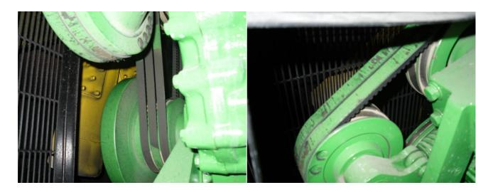
The main fan belts can also be examined from this side, visually check the parts of the belts that can be seen and check they appear to be in good condition with no cracking. There are 3 belts driving the main radiator fan, and the 2 that drive the water pump, make sure they are present. The green paint on the belts is unimportant but the belt condition under the paint is important.
