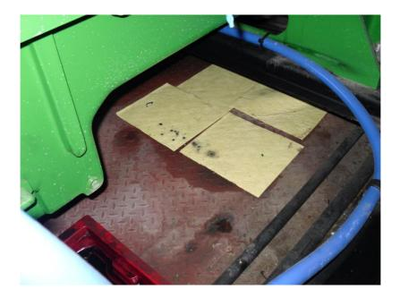
The main floor under the generator should also be checked at this time for any fluids that might have leaked from any pipe work, this could include diesel oil, engine oil, cooling water, if anything abnormal is found this should be investigated further. Pay special attention to under the main cooling radiator at the front of the engine, any loss of coolant could result in major problems when the generator set is running.
