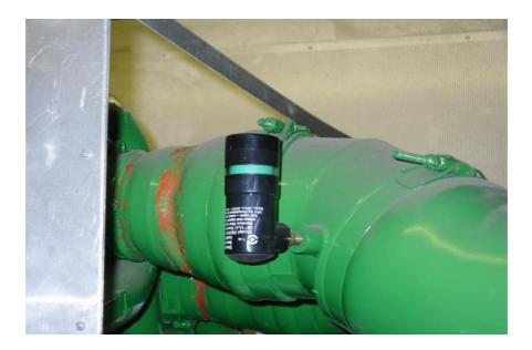
Slightly further along is the second of the two air intake suction gauges to check, as before this should show a *green* band.
