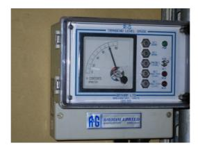
The main fuel tank of 5000 litres has a level gauge that is situated in the electrical cabin next to the generator.
