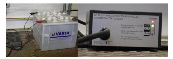
The spare standby batteries should be checked to make sure the float charger is working. One red power light and one Green light indicating the battery is fully charged and being float charged. The electrolyte levels on all cells (12 in total, 6 on each battery) should be checked by removing the tops and visually checking for the electrolyte level to 15mm above the plates inside and if needed toped up with distilled water. **NEVERADDACID**. Check also that no cell is gassing excessively.
