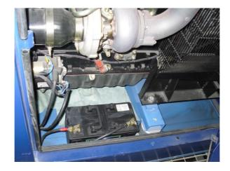
The battery checks are the same as the Corsham Street generator but a screwdriver will be needed to lift of the protective cover on the cells to view the electrolyte level, note there is only one 12V battery on this generator. The floor of the generator can be checked for leaking fluids.
